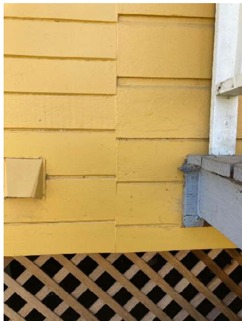
Figure 7- Siding transition, North Elev. Original on right. 2024, author photo.
