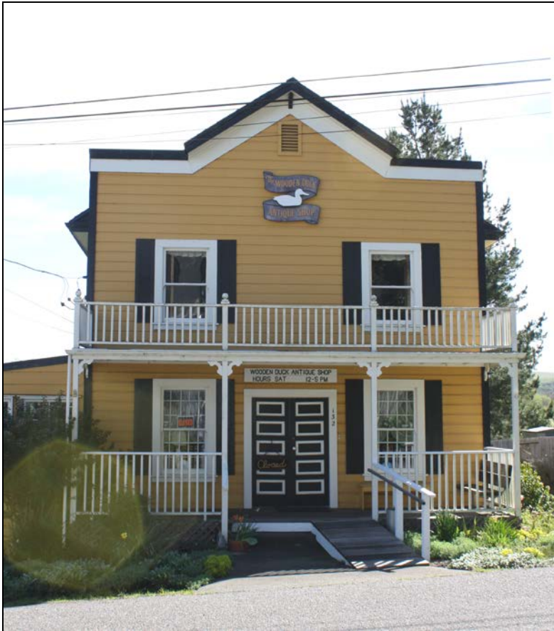
Front (west) facade
