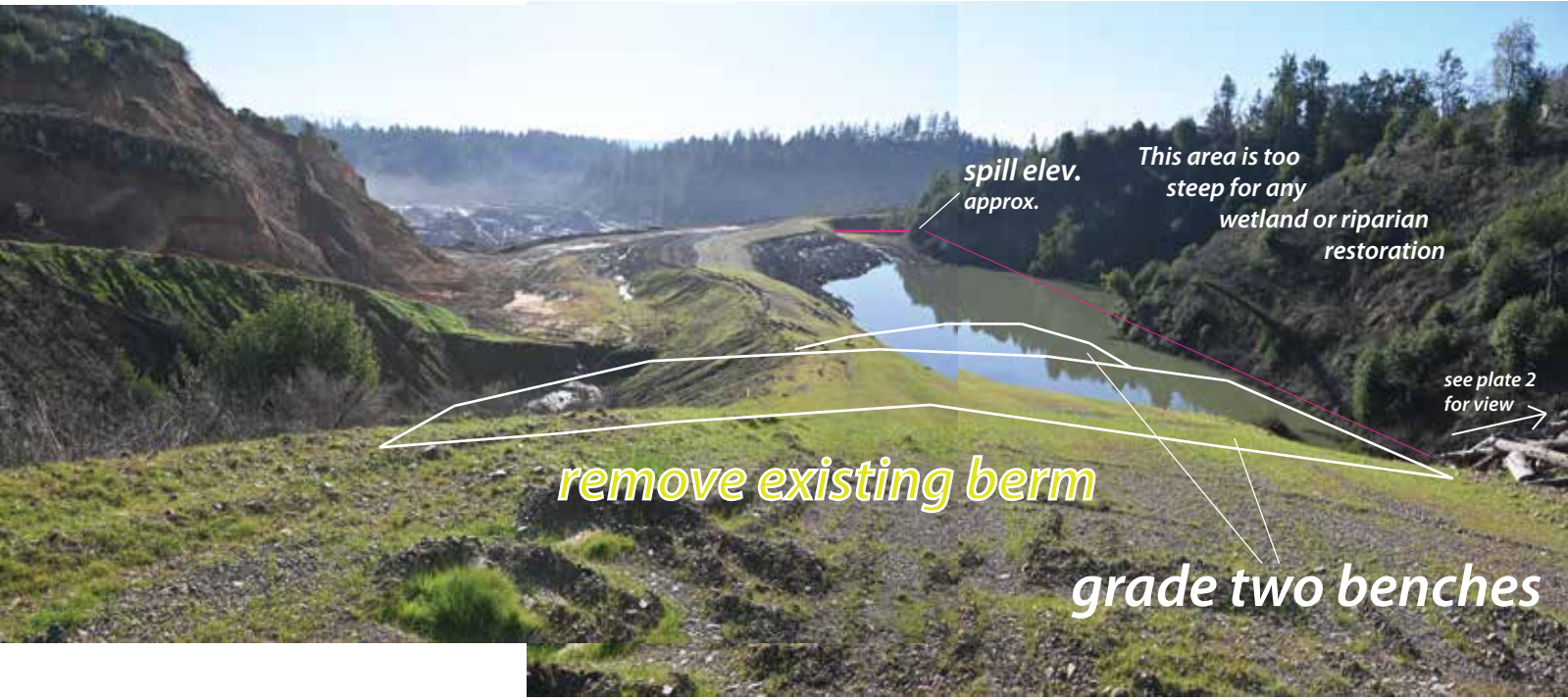
Plate 1. Looking south across reclamation area, showing existing pond and berm. After removal of the berm and reconnection of the small watershed area (to the left), two level benches would be graded roughly as shown above, at approximately three and five feet below the pond's spill elevation. Canyon Rock Quarry, Forestville; February, 2025.
