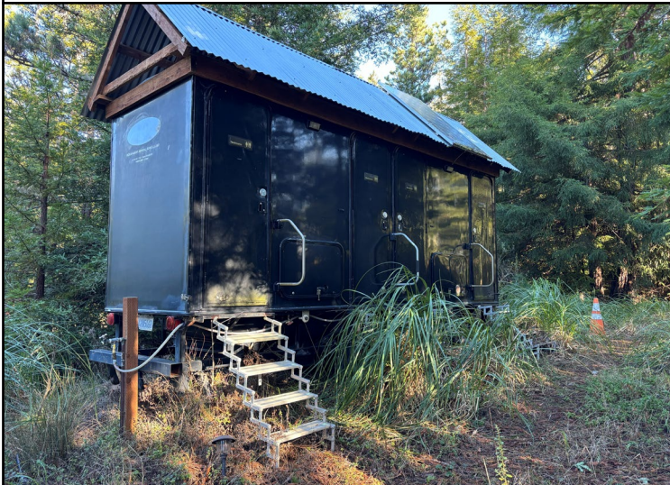
Photo 3: One of the existing restroom facilities within the Ruderal/Developed portion of the Study Area.
