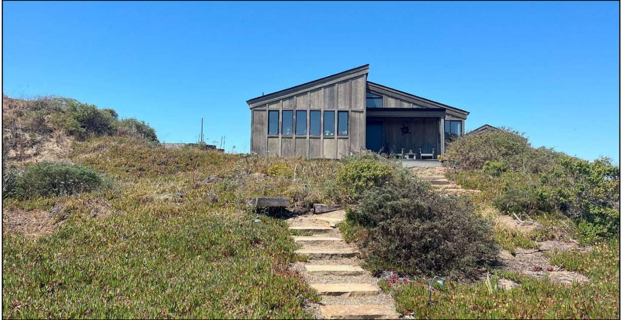
Existing single-family residence, the subject of the proposed project. Note existing development (e.g., stairs, residence) and iceplant mats in the foreground.
