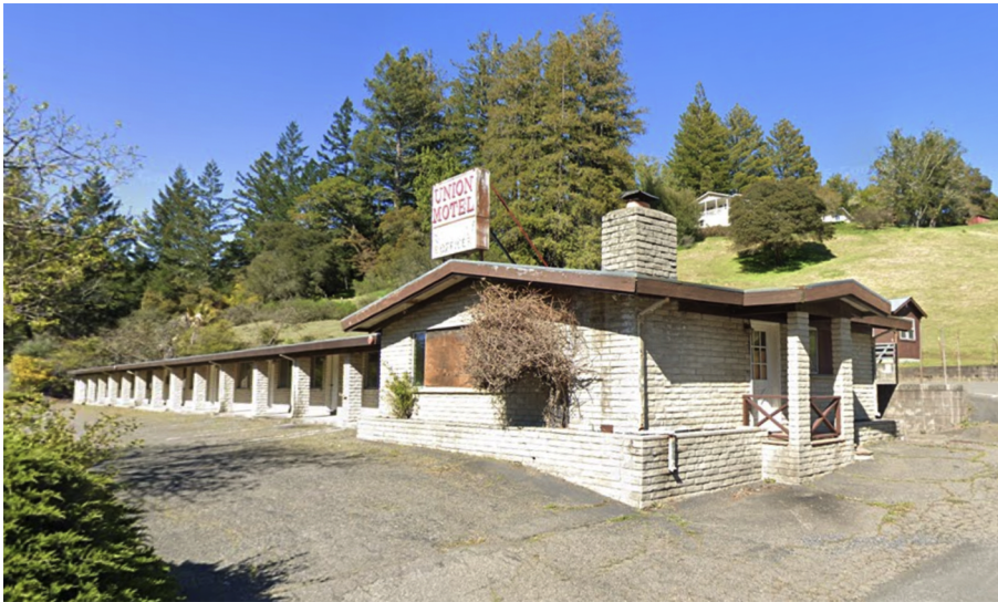
6 - MOTEL LOOKING NORTHEAST
