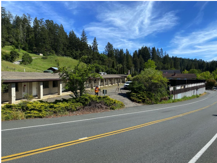
1 - MOTEL & POOL STRUCTURE LOOKING SOUTH
