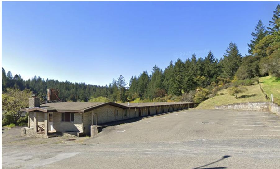
7 - MOTEL LOOKING NORTHWEST
