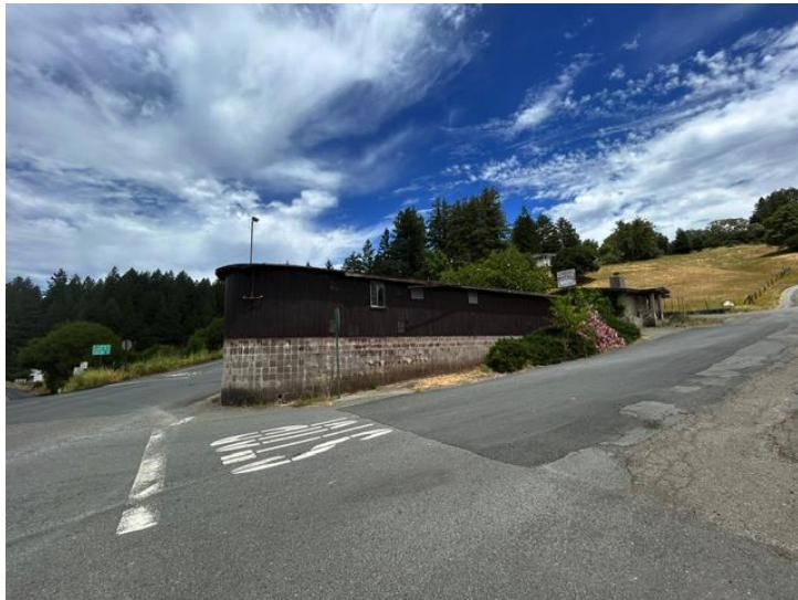
3 - POOL STRUCTURE LOOKING NORTH
