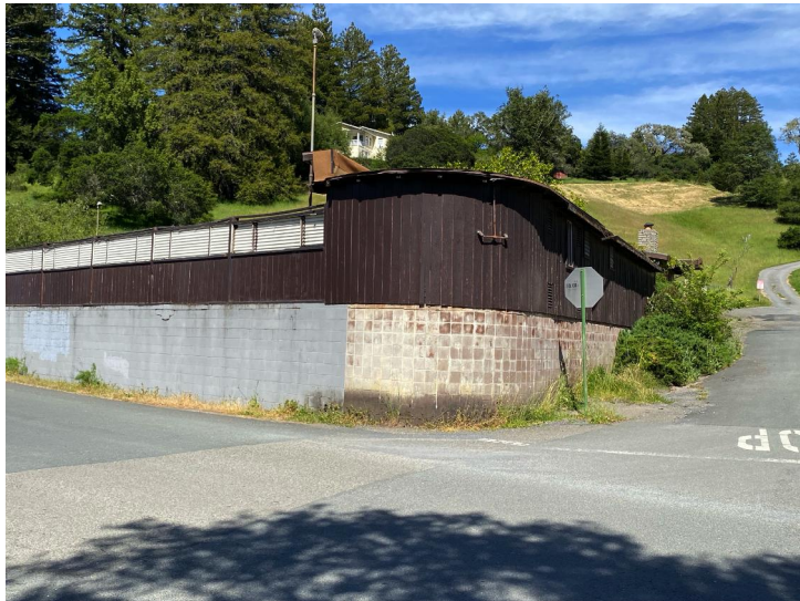
3 - POOL STRUCTURE LOOKING EAST
